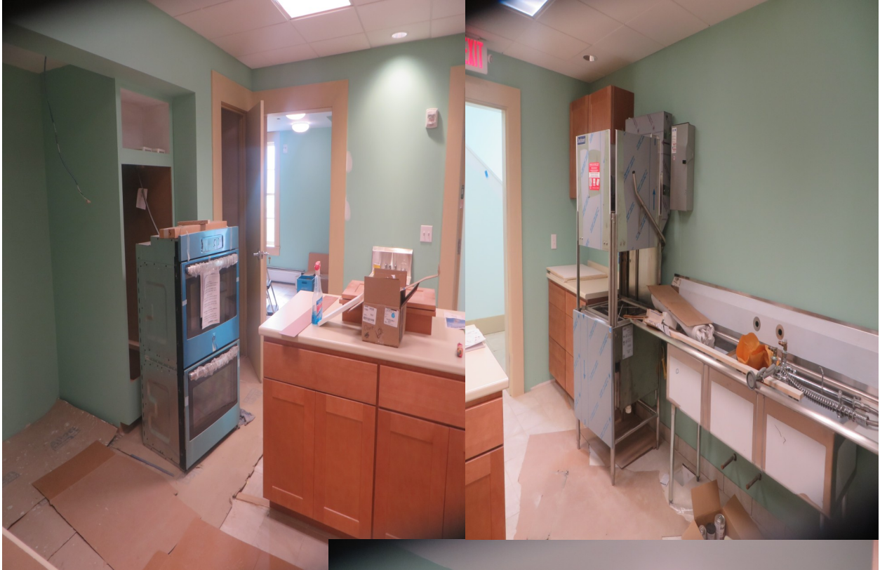
The kitchen and bathroom starting to take shape
