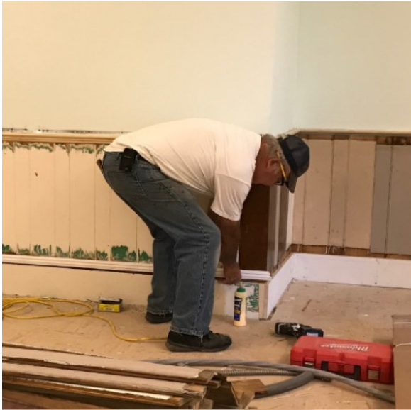
Stanley replacing the wainscoting and painted
