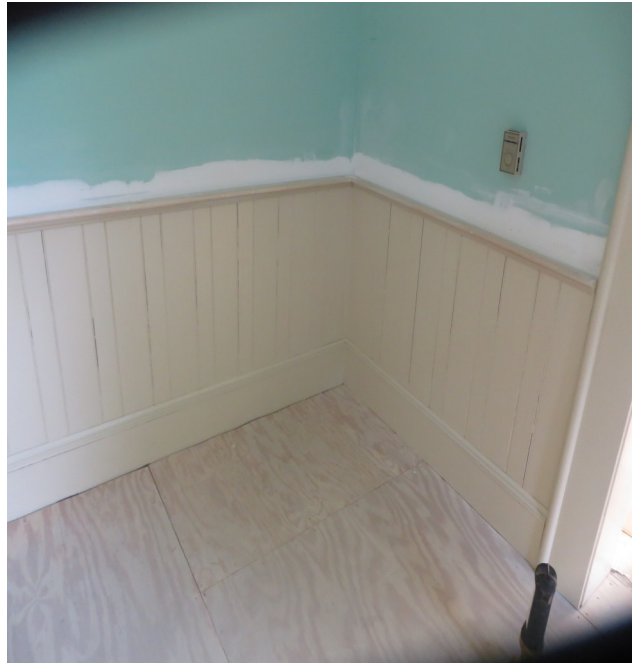
Stanley replacing the wainscoting and painted
