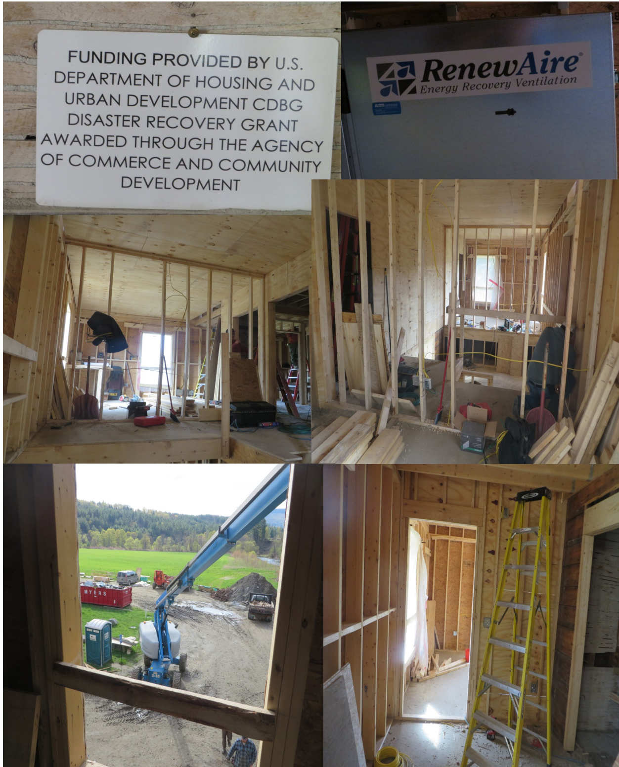
All in the new addition
