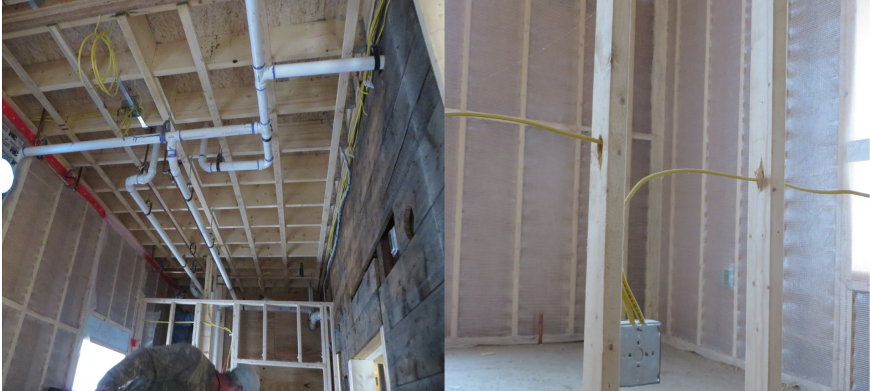
Piping and wiring in the new addition
