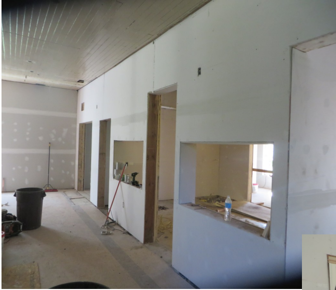
Sheetrock on walls outside kitchen
