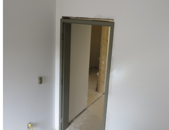
Door jambs installed
