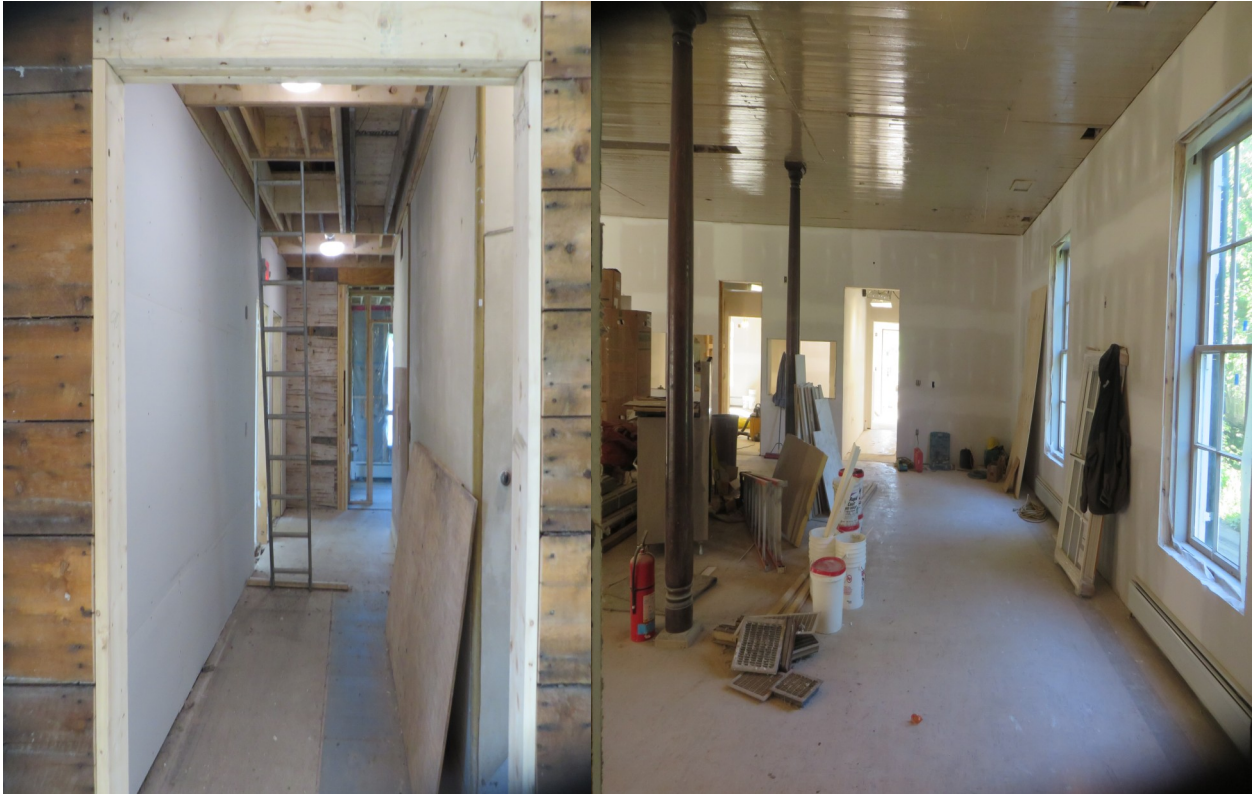
Looking down the hallway on the second floor
