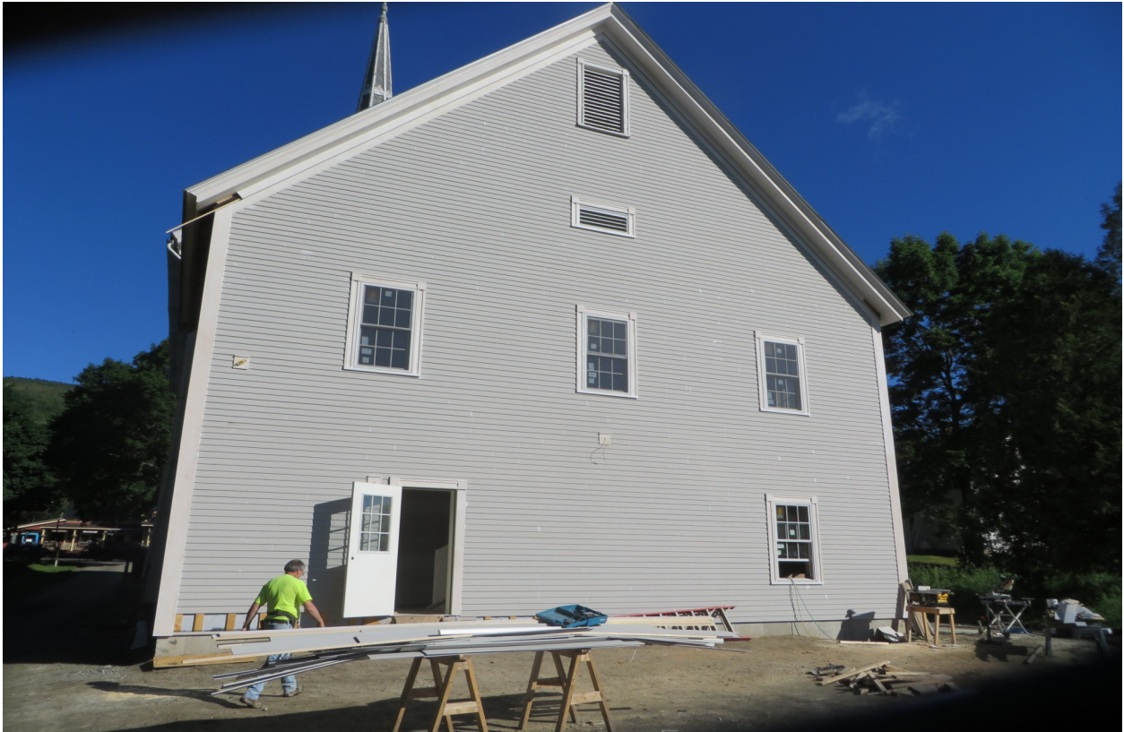
Siding being completed
