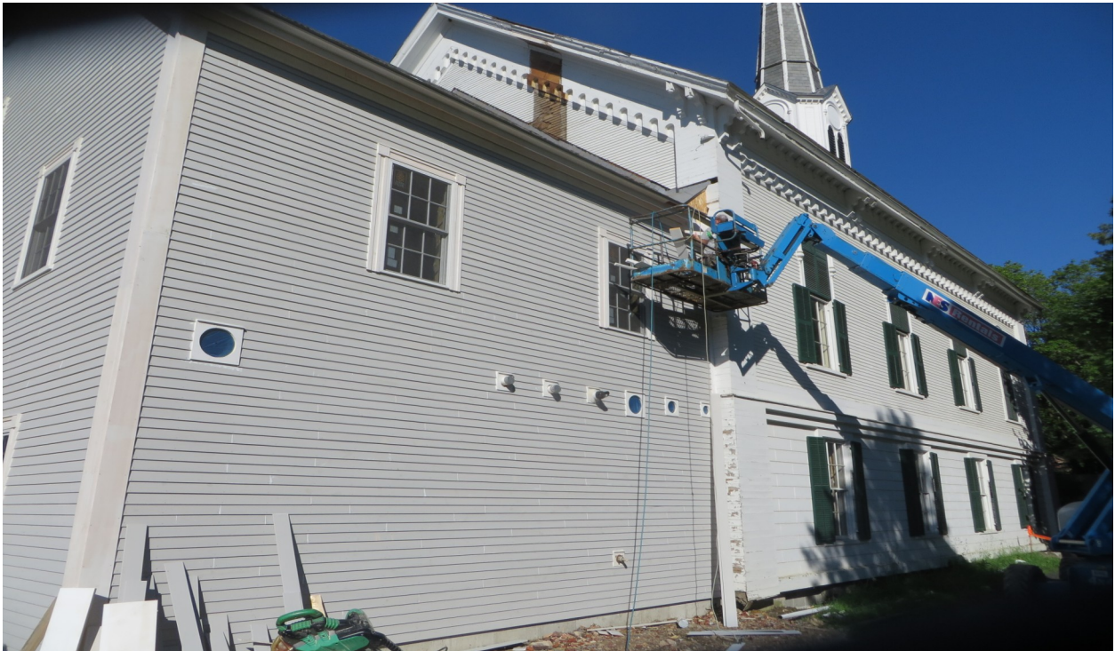
Siding being completed
