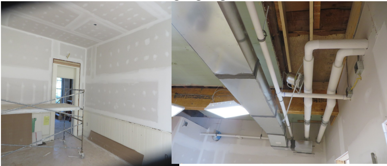
Drywall taped and mudded
