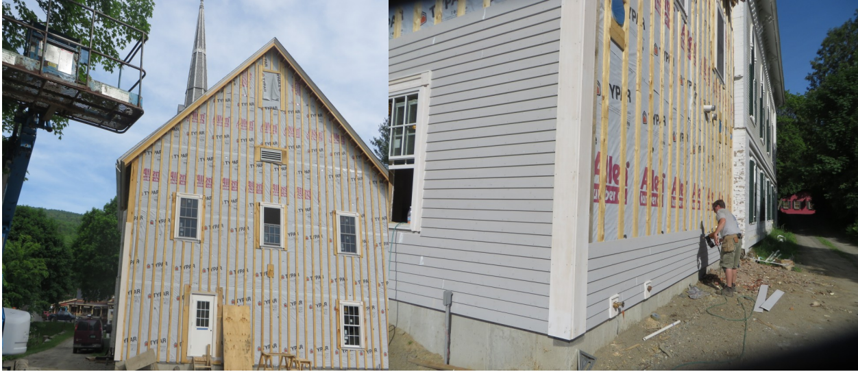
Siding is going on
