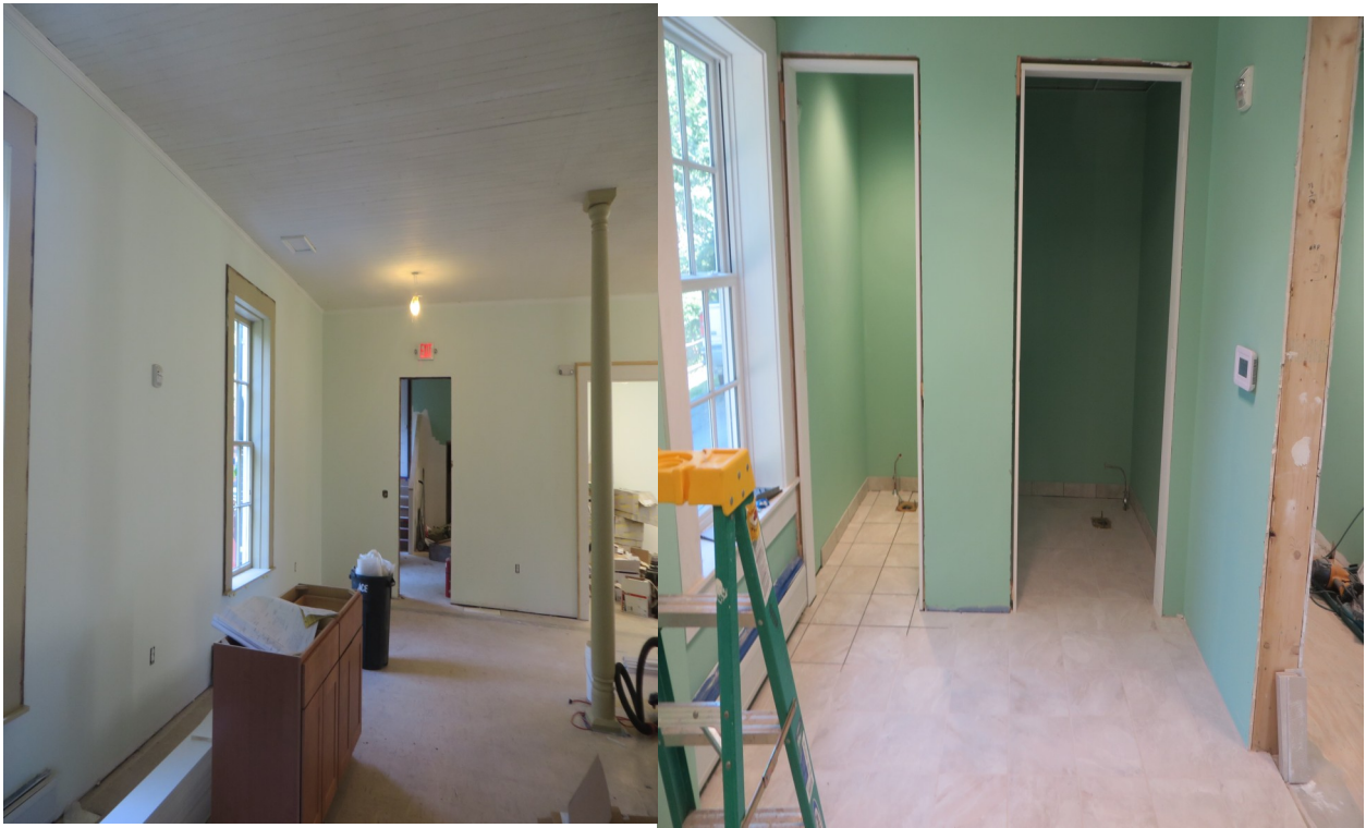
Dining room walls & ceiling painted and bathroom floor & painting done
