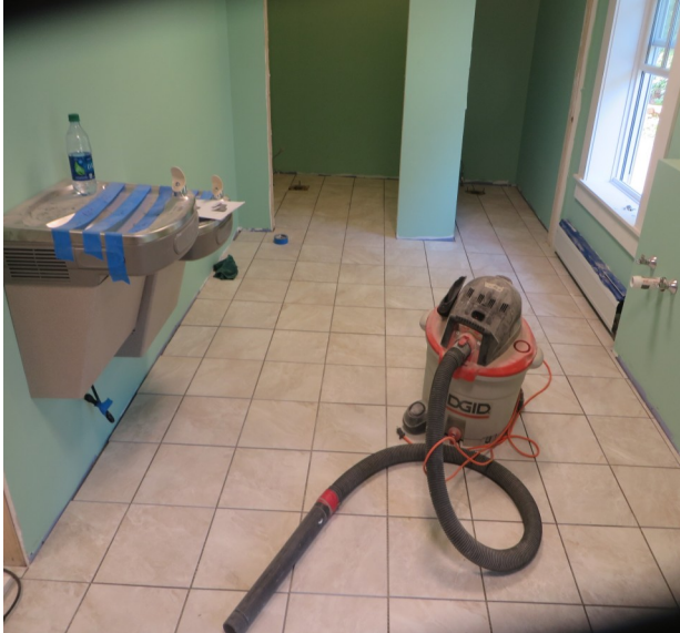
New bathroom floor
