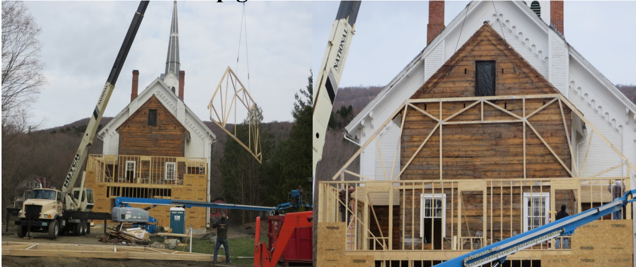
Up go the Roof Trusses
